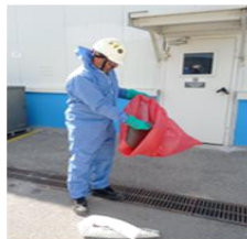
Absorbent cloth and sausage surrounding the chemical are placed in a contaminated waste bag
