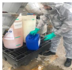
Personnel raise the chemical canister upright to prevent further spillage
