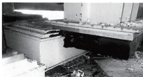
Fig.1 The photograph of the broken rubber bearing by the Great East Japan Earthquake<sup>1)</sup>.
