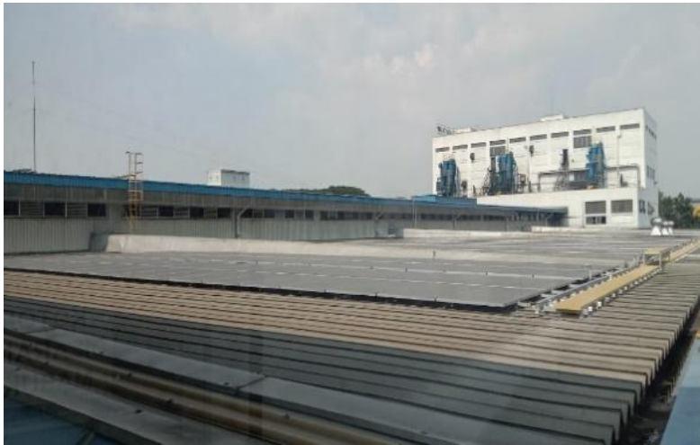
Solar Panels of Energy source
