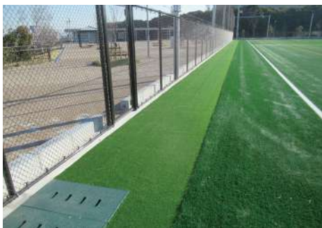
Reducing wind-blown dispersion by installing permeable artificial turf as a filter material over rainwater gutters and surrounding the perimeter with blocks
