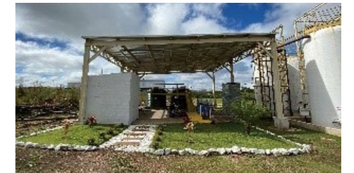
Wastewater recycling facilities (Brazil Factory)
