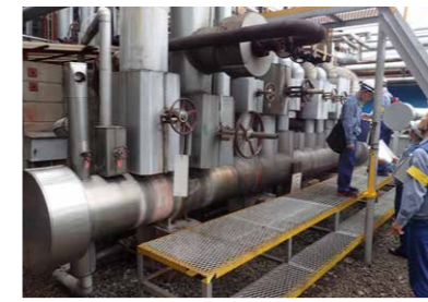
Steam pipe header survey (Shirakawa Factory)
