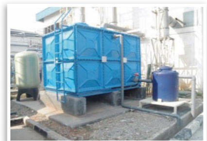
Rainwater tank (Indonesia Factory)
