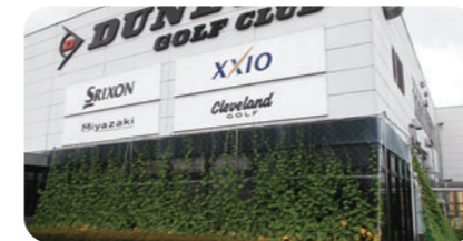
A large green curtain was constructed along the office building of the factory.
