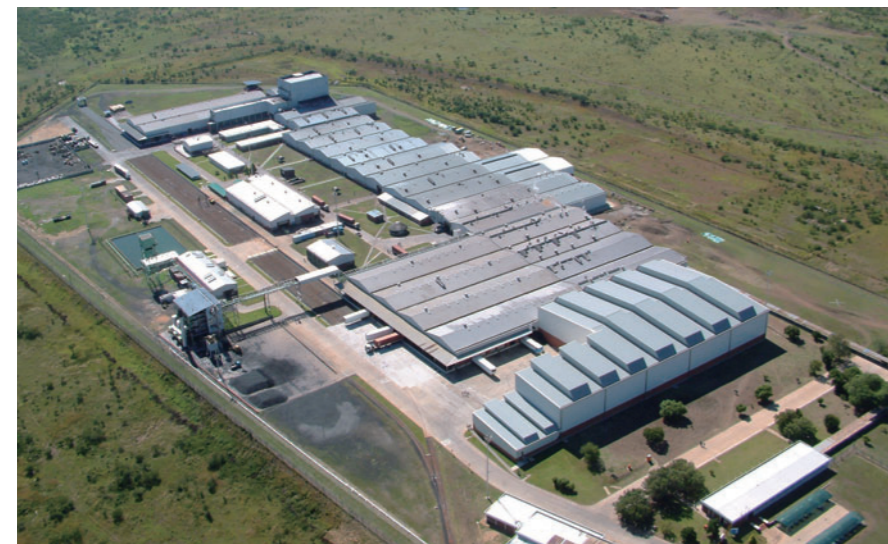
Bird's-eye view of the South Africa Factory
