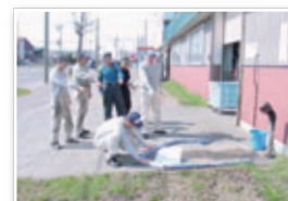
Carrying out leak tests to prevent environmental pollution
