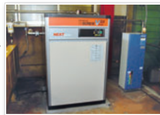
Newly installed screw compressor and drain master (for separating oil and water)
