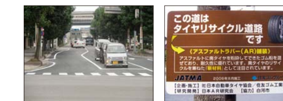
A road paved with asphalt-rubber in Shirakawa City
