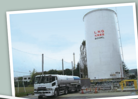
One of Japan's largest natural gas satellites to be built at Shirakawa Factory
